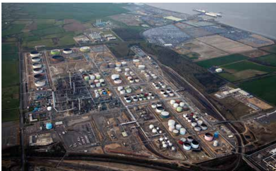
At the end of 2019 TLOR will begin work on its next project – improving the product quality of the facility’s HDS3 unit
