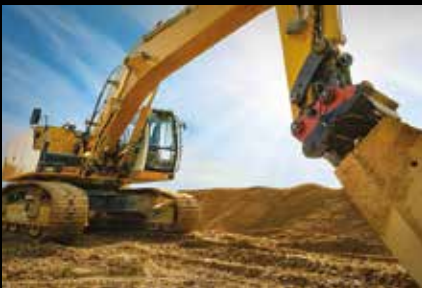
GAS OIL CONDITIONER
