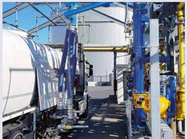
Carbis Loadtec LA210 bottom hose loading skid
