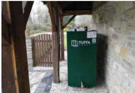
**1100L steel bunded oil tank compatible with HVO and HVO blends**
