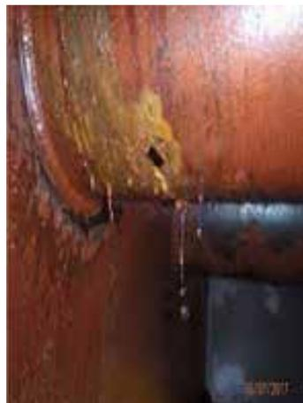
Leaking Pipe, 10 drips a minute = 600l in 6 months!!
