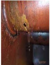
Leaking Pipe, 10 drips a minute = 600l in 6 months!!
