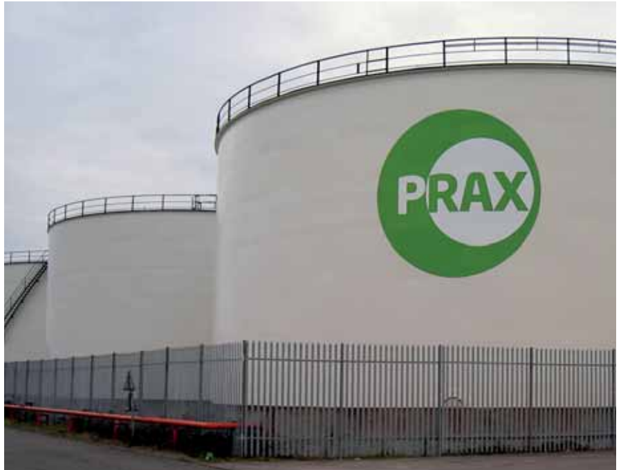
Prax Petroleum – establishing a stronger foothold in the UK fuel supply sector. The company acquired a terminal in Cardiff last year
