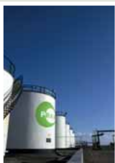
The Prax terminal at Cardiff Docks, which imports product via rail and sea, has a storage capacity of approximately 30m litres.. Products available – kerosene, diesel, and gas oil – can be lifted by road, rail, and sea
