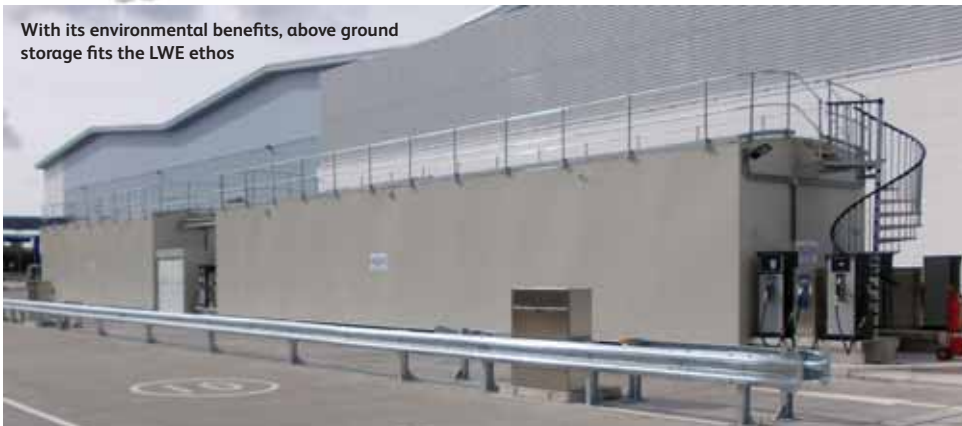
The OTS MultiServ modular filling station – recently deployed at Certas Energy's new Trafford Park depot
