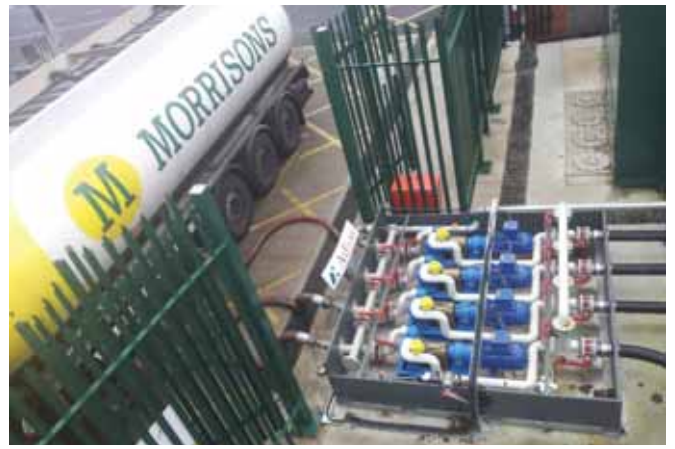
Blackmer sliding vane pumps – used by Berrys for fuel unloading at forecourts
