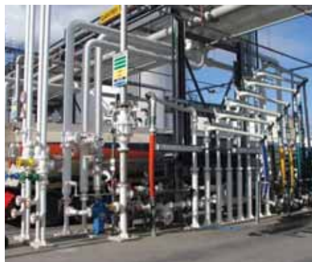
A PDE project for LSS in Derry
