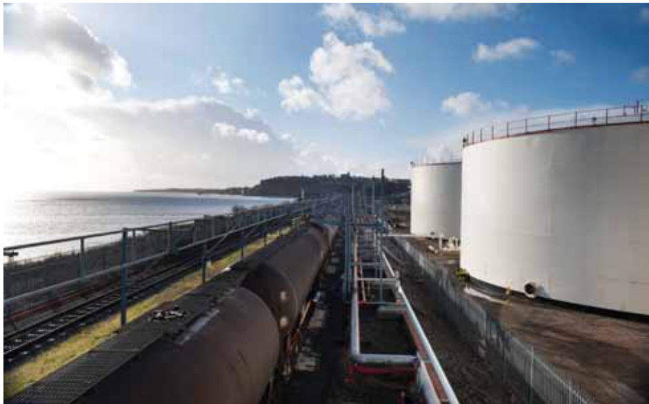
Strategically important to the South Wales and south west region, the Cardiff terminal has seen £10 million invested since 2006
