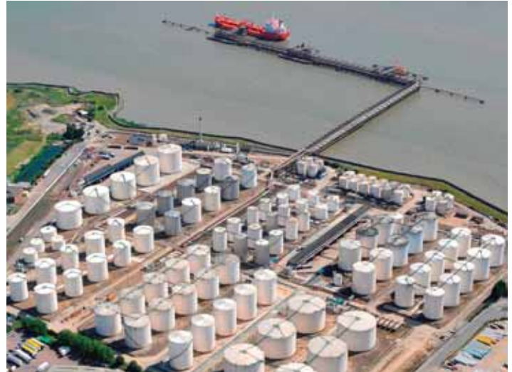
Vopak services the market through three strategically located marine terminals in London (pictured), Teesside and Windmill (South Wales) with a total capacity of 720,000m 3 of storage
