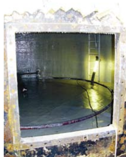
Above ground tank with double skin lining
