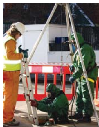
An operative prepares to enter and clean a gas freed below ground tank
