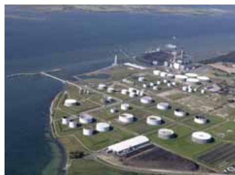
The recently acquired Gulfhavn terminal in Denmark
