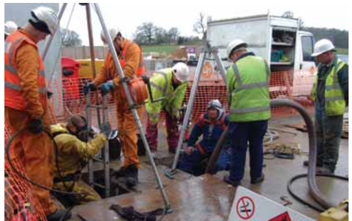
The project to clean and line tanks in full swing
